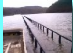
Sleeved timber rails
