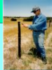
Installing wire clips
