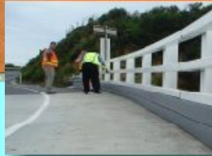
Motorcycle Roadside Safety Barrier
