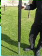
Installing Post Sleeves
