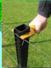
Installing wire clips
